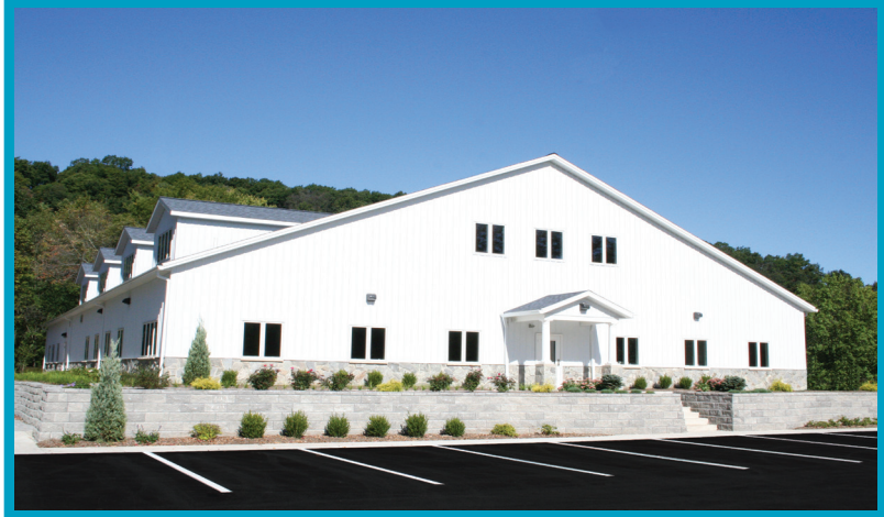
The corporate headquarters of QBC Diagnostics
